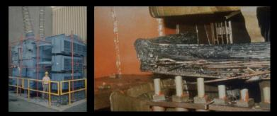
Disrupted transformer after solar storm, Quebec, 1989 Image credit: Eskom, T. Makhosi, G. Coetzee
